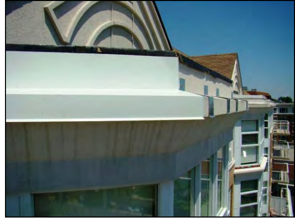
Figure 33: Example of metal flashing at EIFS cornice.
