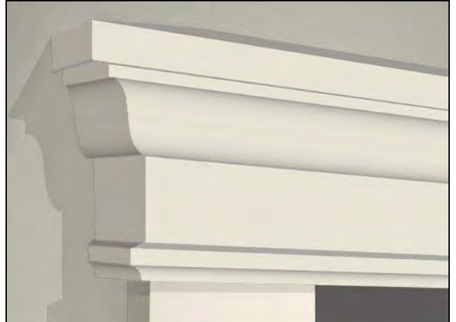
Figure 26: Headers - Mouldings applied over the top of windows or doors. Headers are often larger and protrude further than trims and may include a drip edge to deflect water.
