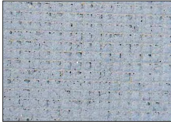
Inadequate Base Coat Coverage
