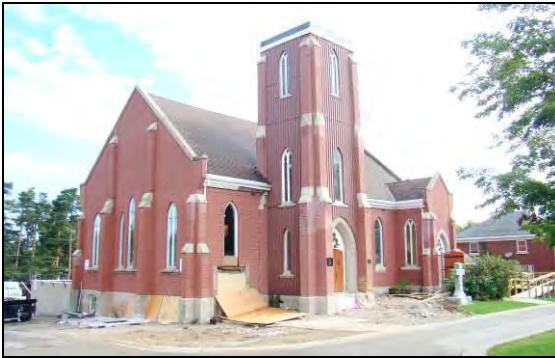
Retrofit – Original Deteriorated Brick
