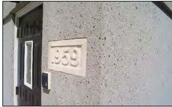
Retrofit – EIFS Simulated Stone Aggregate
