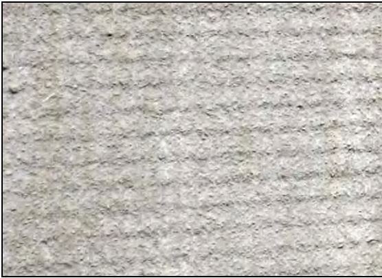
Acceptable Base Coat Coverage
