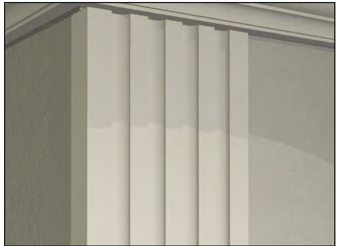
Figure 28: Pilasters - A shallow rectangular column attached to the face of a wall, designed to look like columns embedded in the wall to provide an illusion of support. Often smooth, they may also be fluted. A pilaster will also typically include a moulded cap and base.
