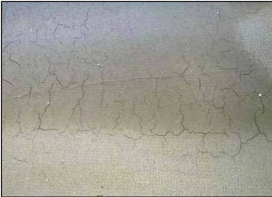
Base Coat Applied Too Thickly
