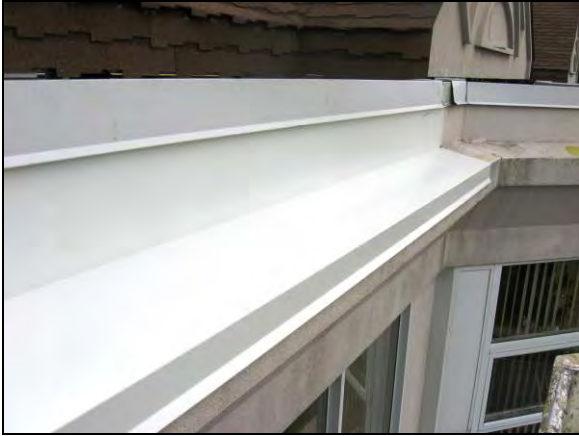
Figure 32: Example of metal flashing at EIFS cornice.
