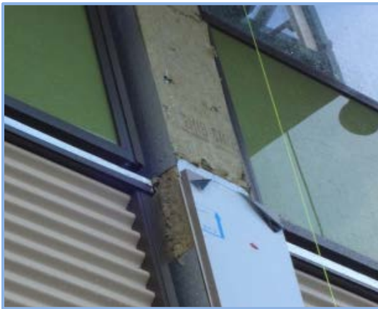
Figure 17: An example of thermal bridging at the interface between assemblies that is NOT captured by wall schedules (not an issue for EIFS)
